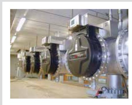
Using a combination of UV light and hydrogen peroxide, the TrojanUVSwiftECT system provides superior disinfection without producing harmful by-products such as bromate.
