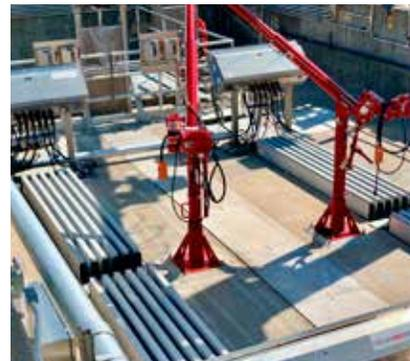
*The TrojanUV3000Plus has a Type 6P rating, making it an ideal option for plants – such as Wastewater Treatment Plant 20 – that are prone to flooding events.*
