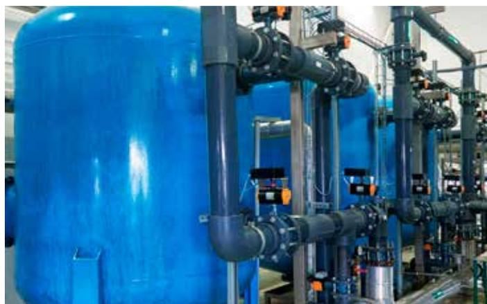
1,4-dioxane breaks through GAC filters more rapidly compared to other contaminants, resulting in reduced filter life and more frequent replacements of media.
