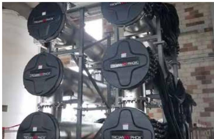
The TrojanUVPhox system in place at the Albert Robles Center uses a UV/ $Cl_2$  approach to UV Advanced Oxidation instead of the more traditional UV/ $H_2O_2$ .
